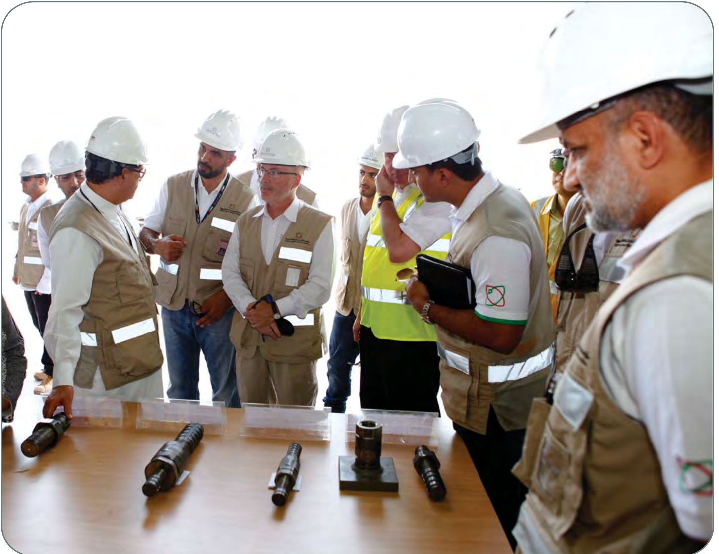
FANR Board Members at the Barakah Nuclear Power Plant review the safety and security measures at the construction site.
