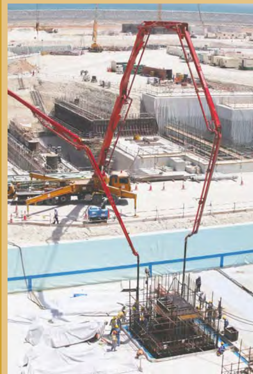
Construction starts for Unit 2 of the Barakah Nuclear Power Plant, May 2013
