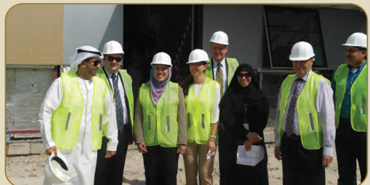
IAEA TC delegation visit to SSDL construction site, Khalifa University campus in Abu Dhabi, 2014
