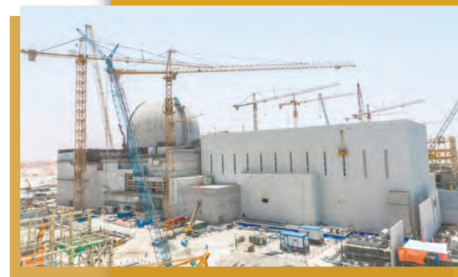
Construction work at Unit 1 of the Barakah Nuclear Power Plant, 2015
