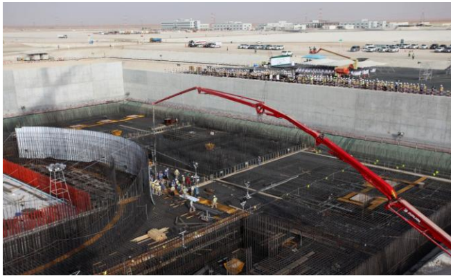
Construction work at the Barakah plant site
