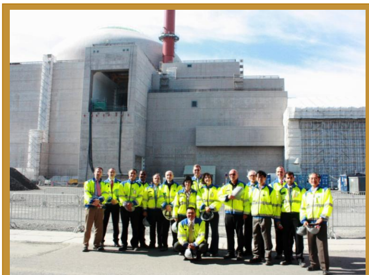
The delegations at the OL3 nuclear reactor construction site
